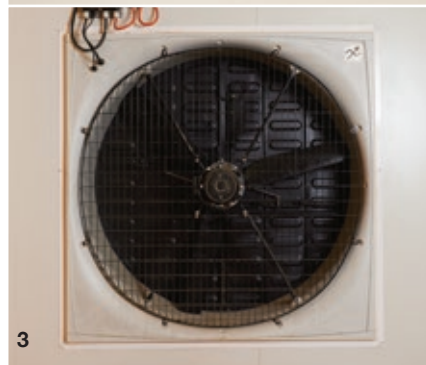
1. Tunnel mode utilises 14 x SKOV BF 50 LPC fans. 2. SKOV mini vent – 164 installed in two sheds. 3. Side wall installed BF50 LPC fan – four per shed. 4. SKOV DA 175 mini vent winch motors.
