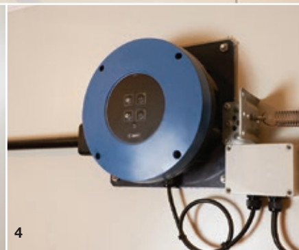
1. Tunnel mode utilises 14 x SKOV BF 50 LPC fans. 2. SKOV mini vent – 164 installed in two sheds. 3. Side wall installed BF50 LPC fan – four per shed. 4. SKOV DA 175 mini vent winch motors.
